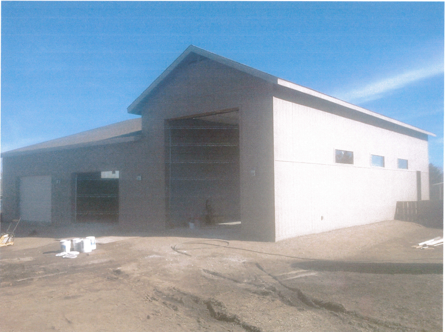
PHOTO 1: WEST & SOUTH SIDES, DOORS FACING WEST EASEMENT.
