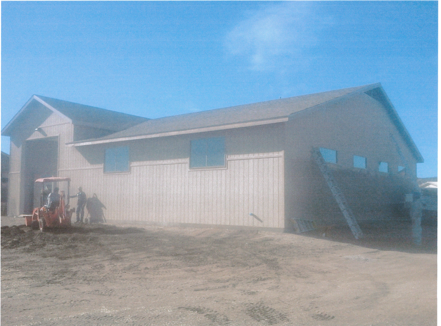
PHOTO 2: EAST & NORTH SIDES.
