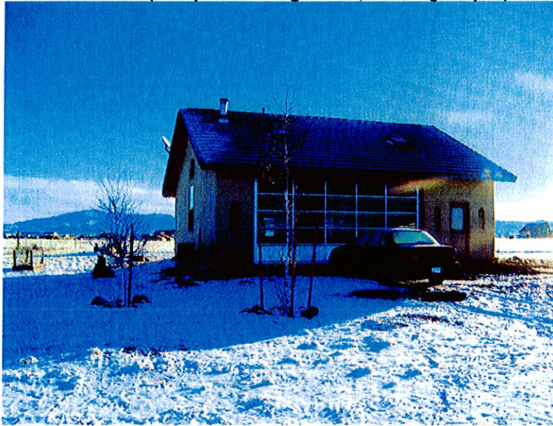
Front View (with partial of Right Side, showing AC pad)
