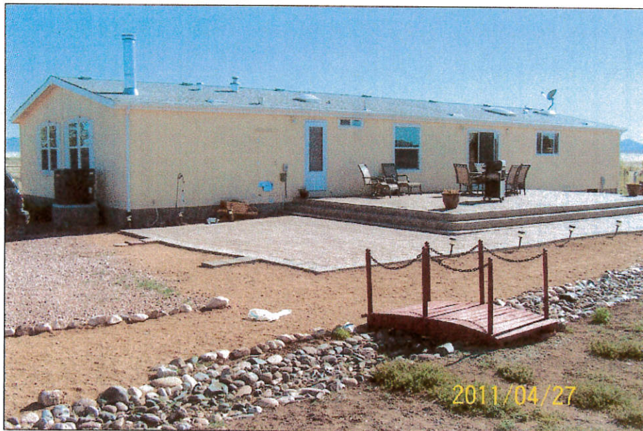
REAR VIEW (from right rear corner))
