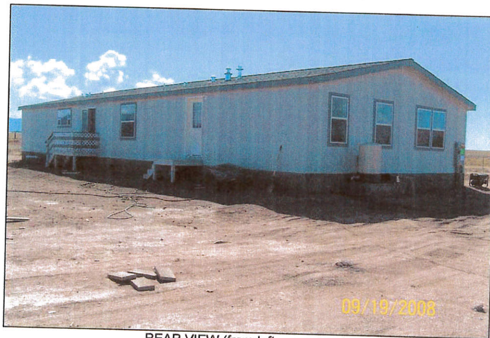
REAR VIEW (from left rear corner)
