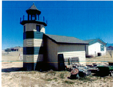
SOUTH AND WEST SIDE SHED LOOKING NORTH 4-14-2014
