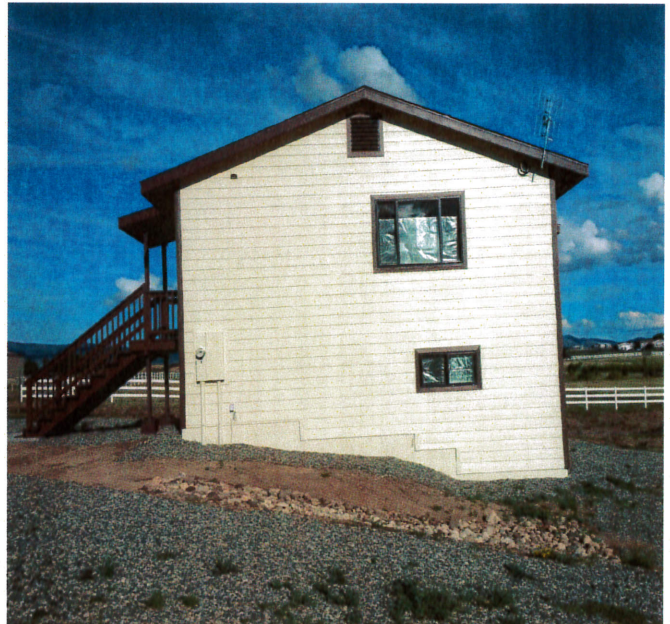
RIGHT SIDE VIEW / WEST SIDE (9-6-2015)
