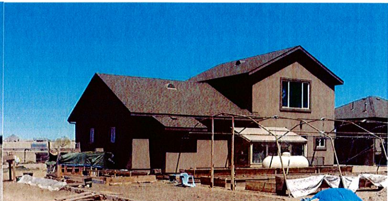
BACK AND WEST SIDE OF DETACHED GARAGE LOOKING NORTHEASTERLY 4-14-2014
