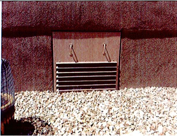
ON EAST SIDE OF HOUSE 4-17-2015
