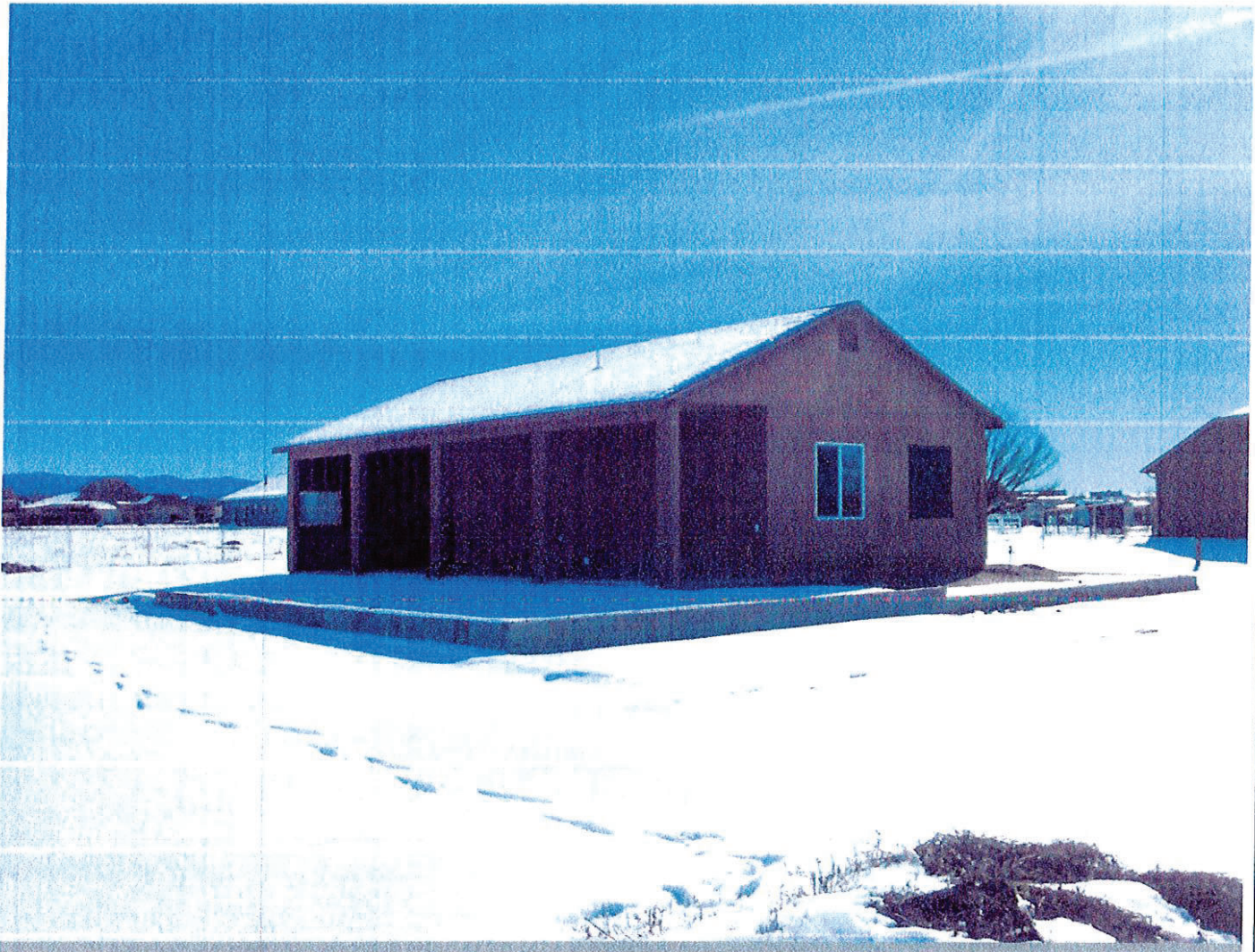
WEST END & NORTH SIDE OF WORKSHOP. C2E ELECTRIC SOCKET AT MID-BUILDING
