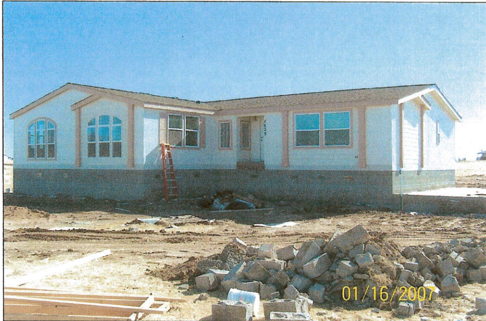
FRONT VIEW (FROM FRONT RIGHT CORNER)
