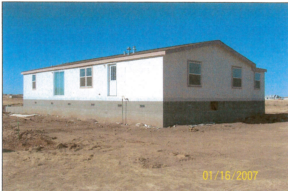
REAR VIEW (FROM LEFT REAR CORNER)
