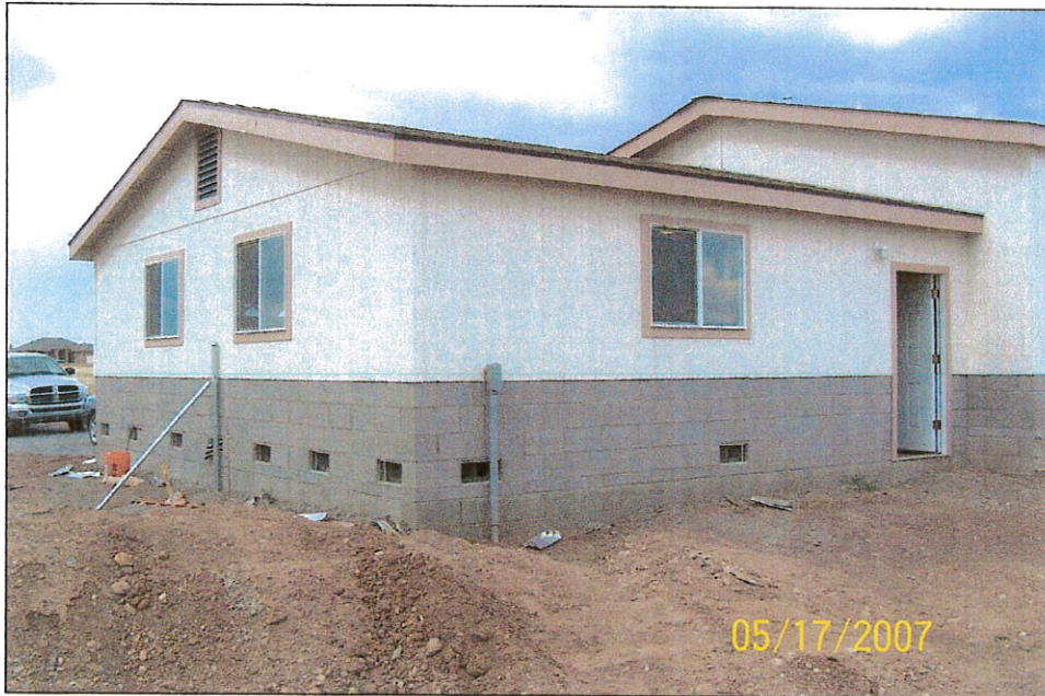
REAR VIEW (FROM RIGHT REAR CORNER)
