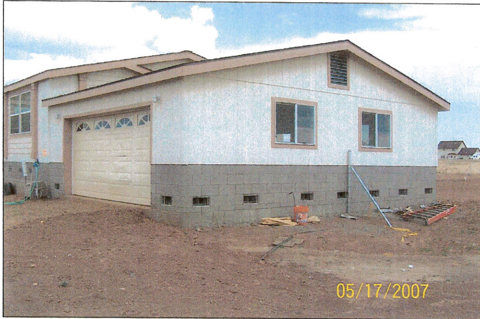
FRONT VIEW (FROM FRONT RIGHT CORNER)
