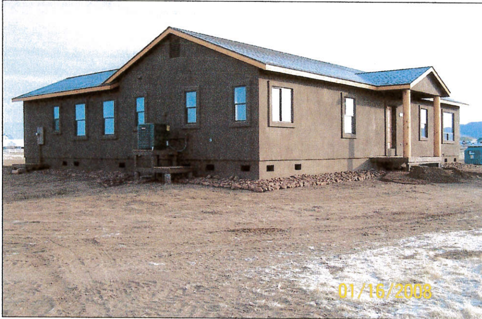
FRONT VIEW (FROM FRONT LEFT CORNER)
