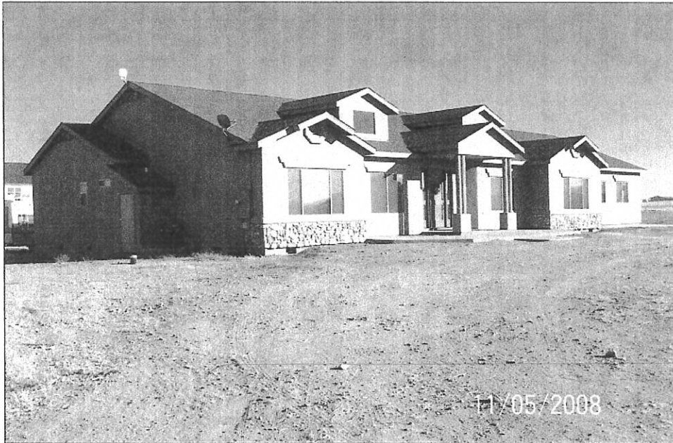
FRONT VIEW (FROM FRONT LEFT CORNER)
