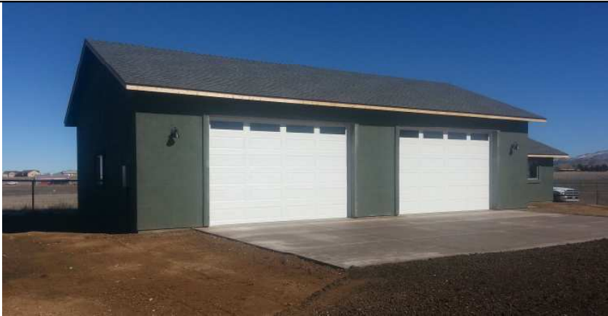
WEST AND SOUTH SIDE LOOKING NORTH FROM ROAD 2-5-2016
