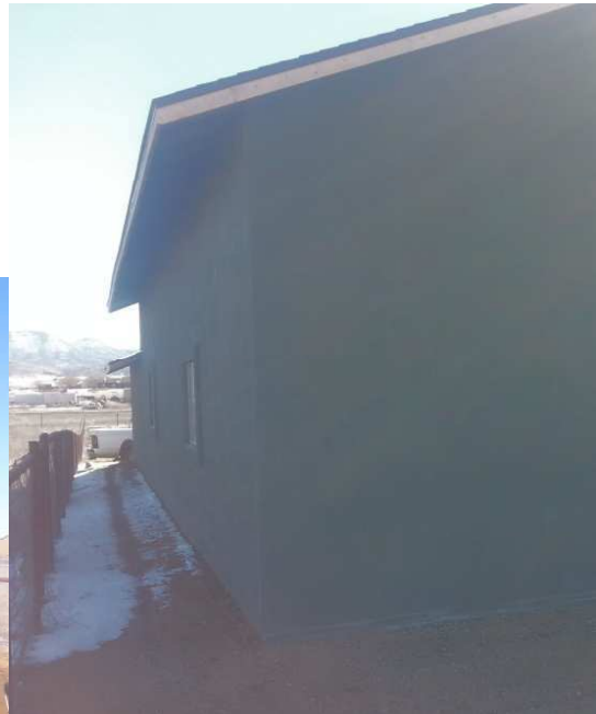
REAR AND NORTH LOOKING EAST 2-5-16
