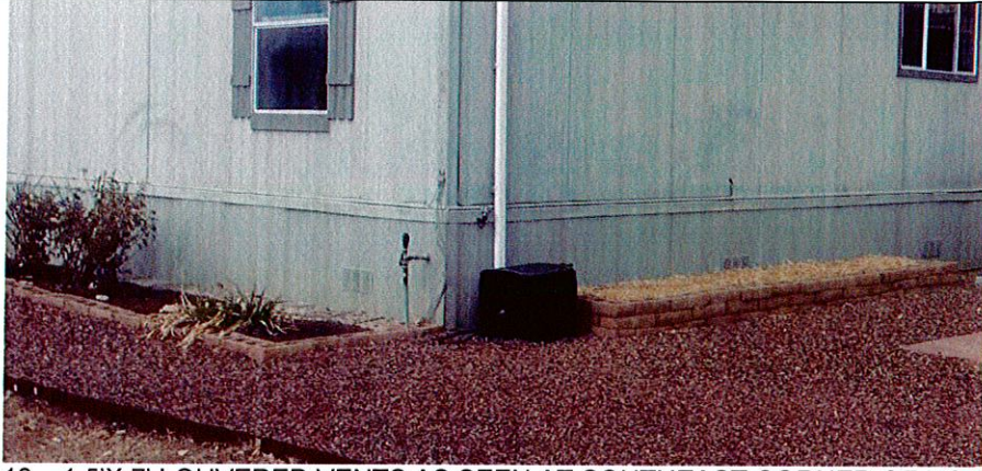
12 - 1.5'X.7' LOUVERED VENTS AS SEEN AT SOUTHEAST CORNER OF HOME 2-03-2014
