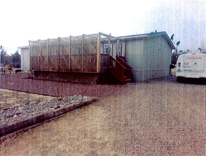
REAR AND NORTH END HOUSE LOOKING WEST
