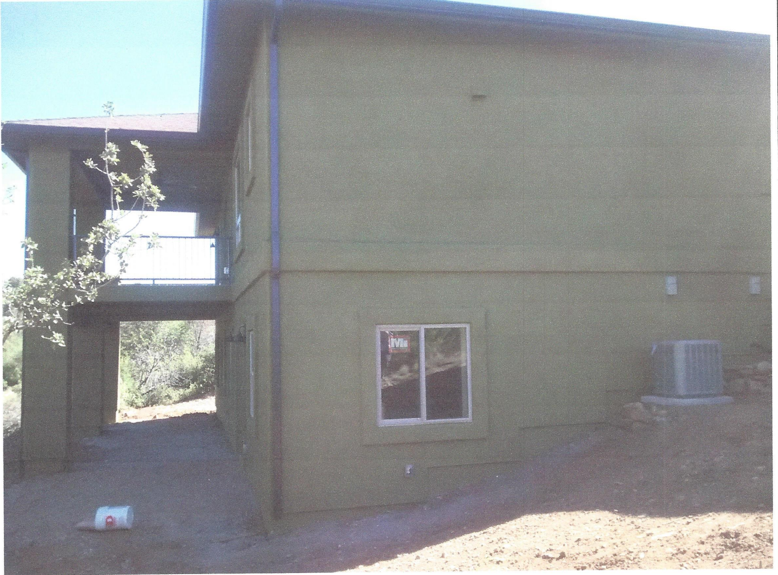
NORTH & EAST SIDES. C2E ON AC PAD. – 7-10-15
