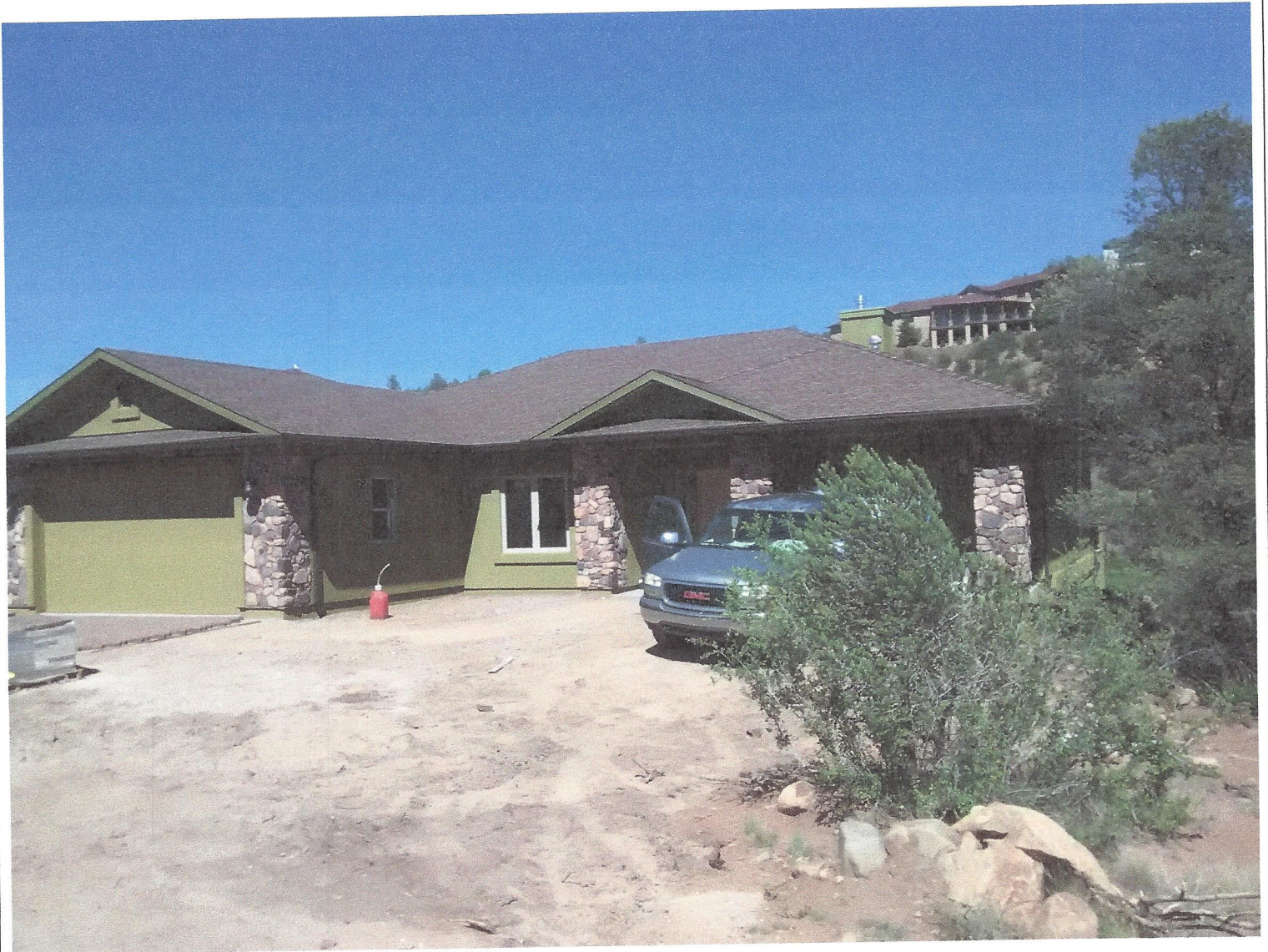
SOUTH AND WEST (STREET) SIDES OF RESIDENCE – 7-10-15
