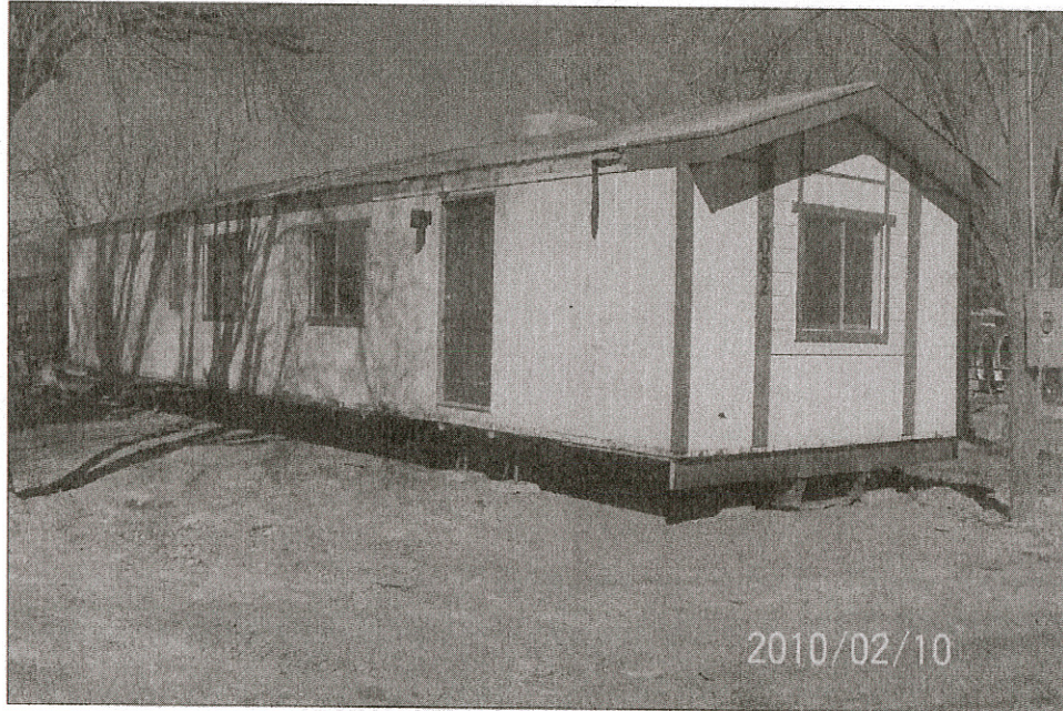
FRONT VIEW (from right front corner)
