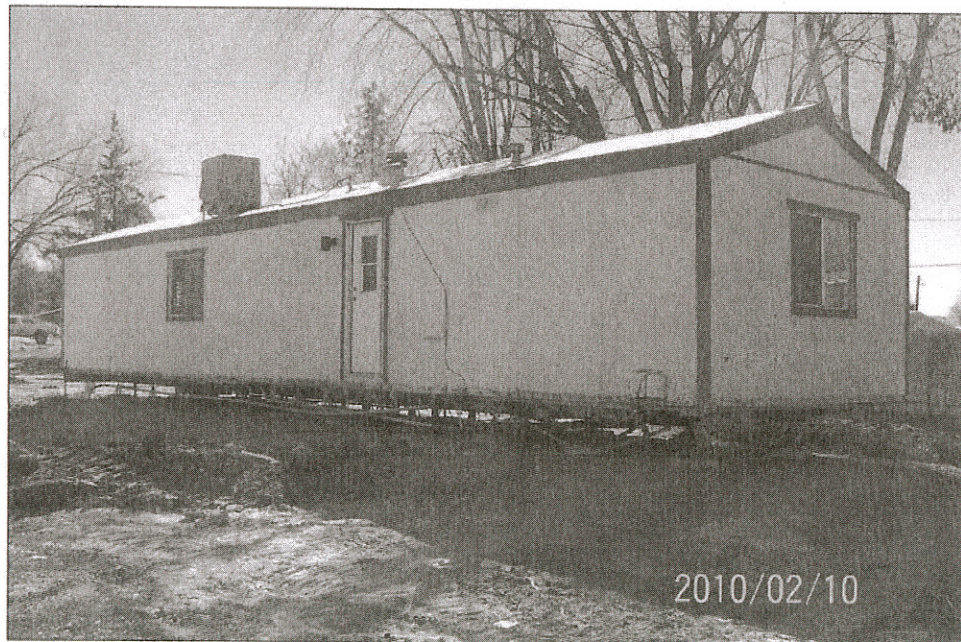
REAR VIEW (from left rear corner)
