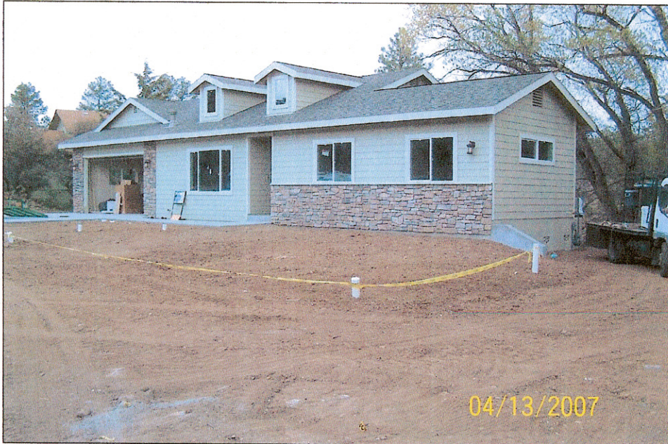
FRONT VIEW (FROM RIGHT FRONT CORNER)
