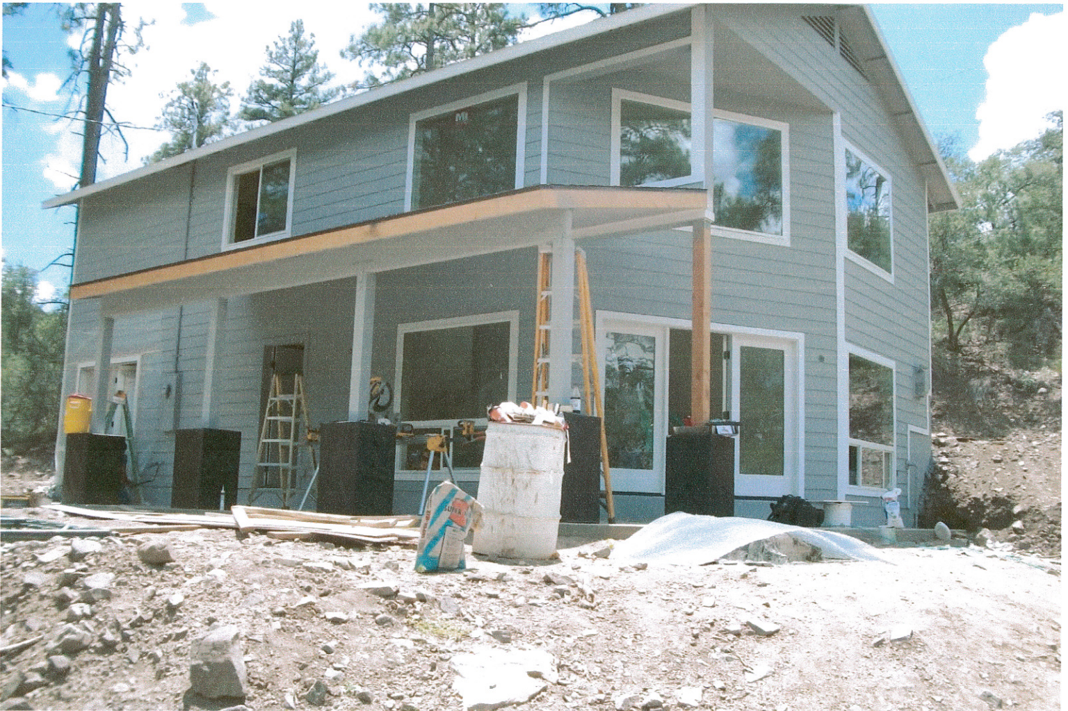
PHOTO 1 : EAST (STREET) SIDE – FRONT YARD
