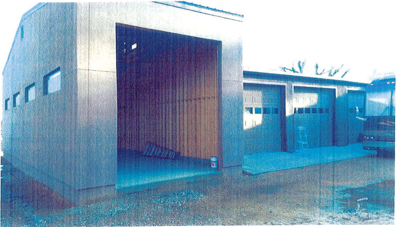
WEST END – SOUTH SIDE FACING ROAD
