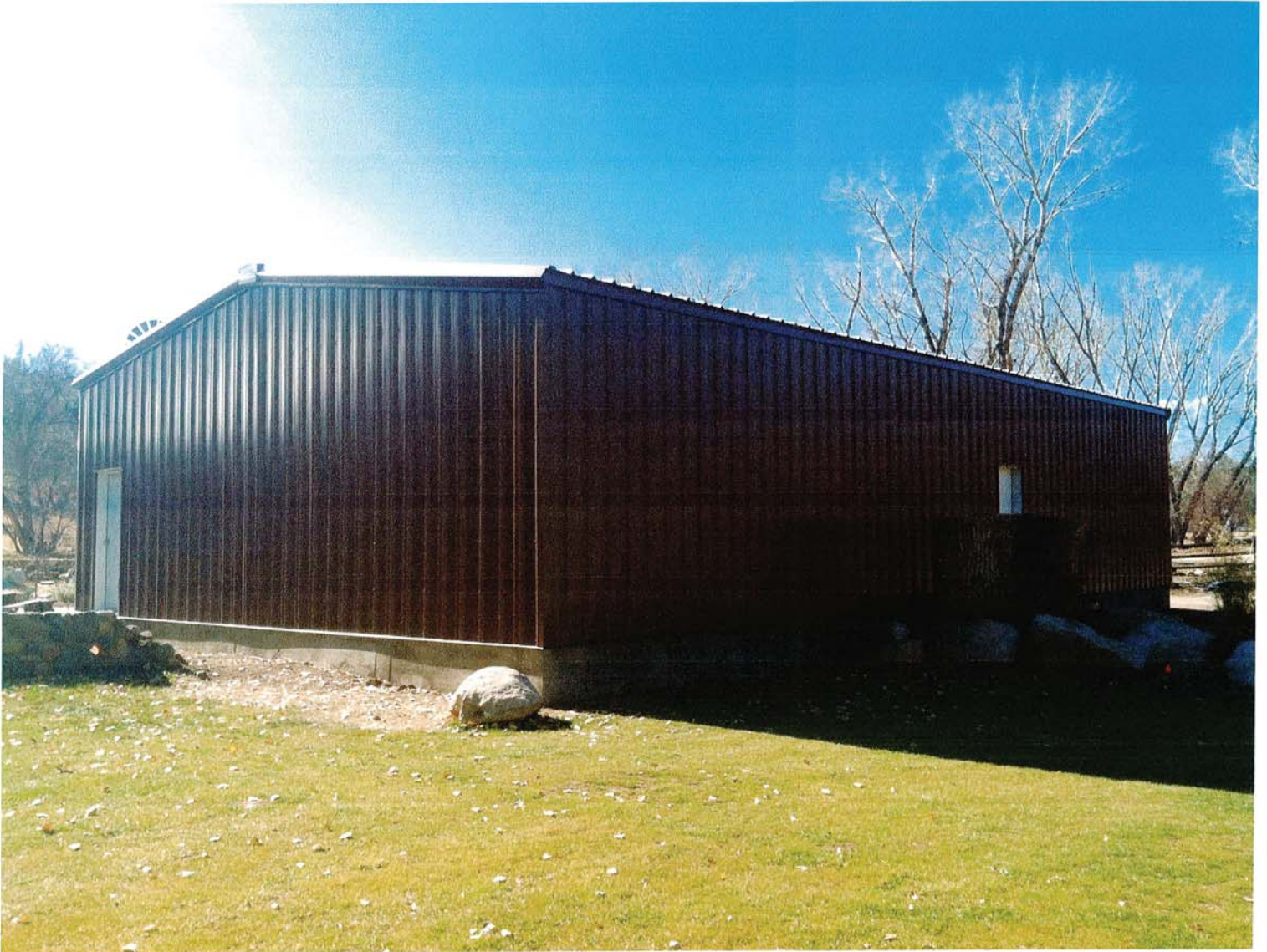
EAST END – NORTH SIDE FACING DRAINAGE
