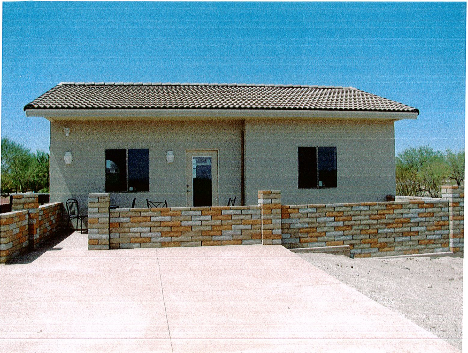
PHOTO NO. 1: EAST SIDE (FRONT) OF RESIDENCE
