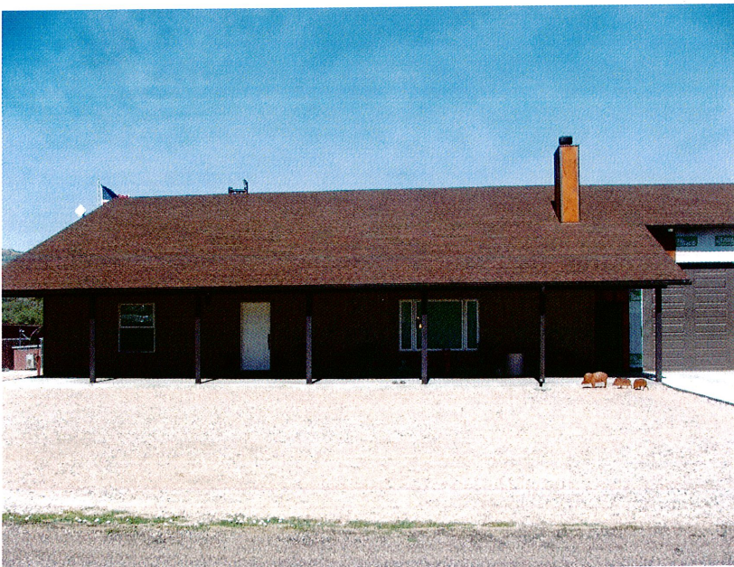
FRONT VIEW (EAST SIDE) OF CONSTRUCTED HOUSE TAKEN 6-02-2013
