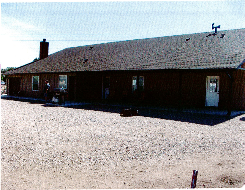
REAR VIEW (WEST SIDE) OF CONSTRUCTED HOUSE TAKEN 6-02-2013
