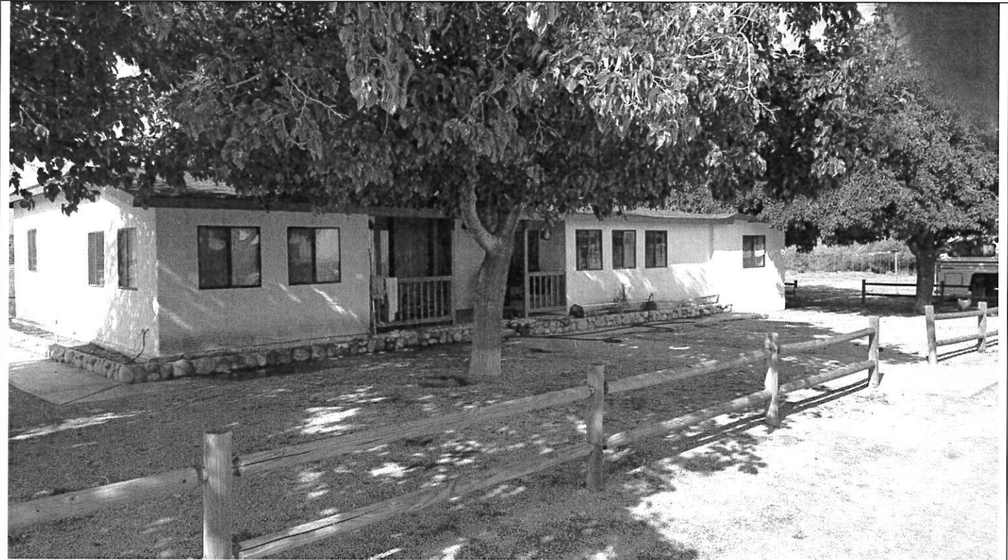
South side of house, front face.
