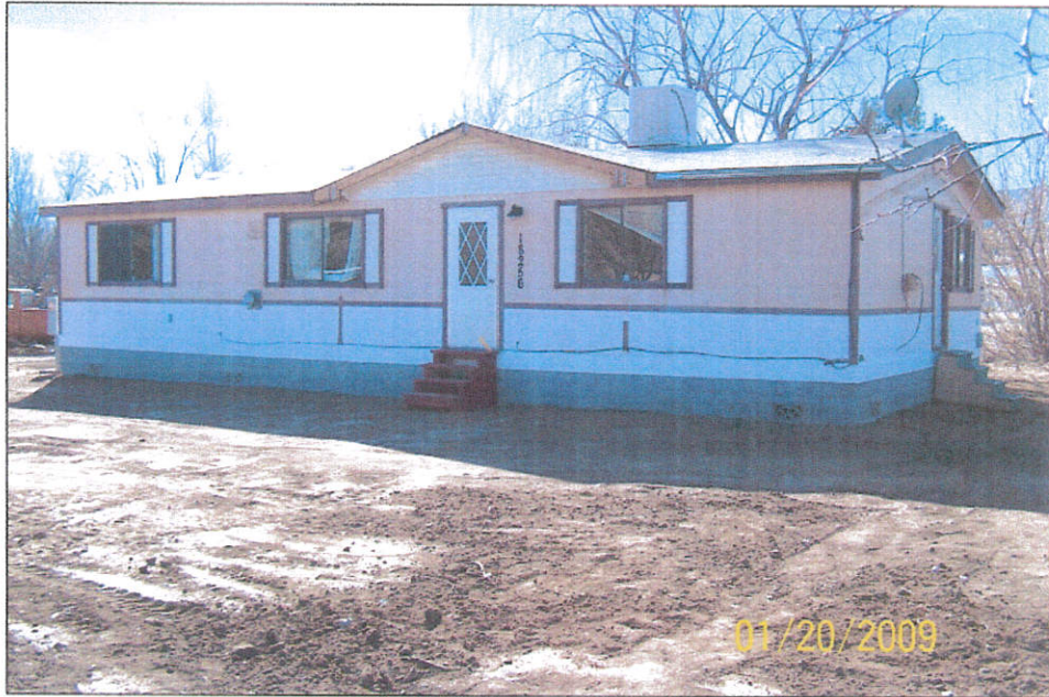
FRONT VIEW (from right front corner)
