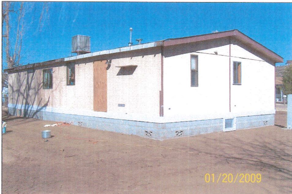
REAR VIEW (from left rear corner)
