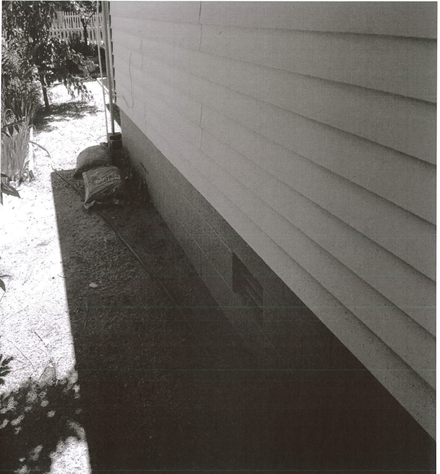
Flood opening in the stem wall, East side of the house
