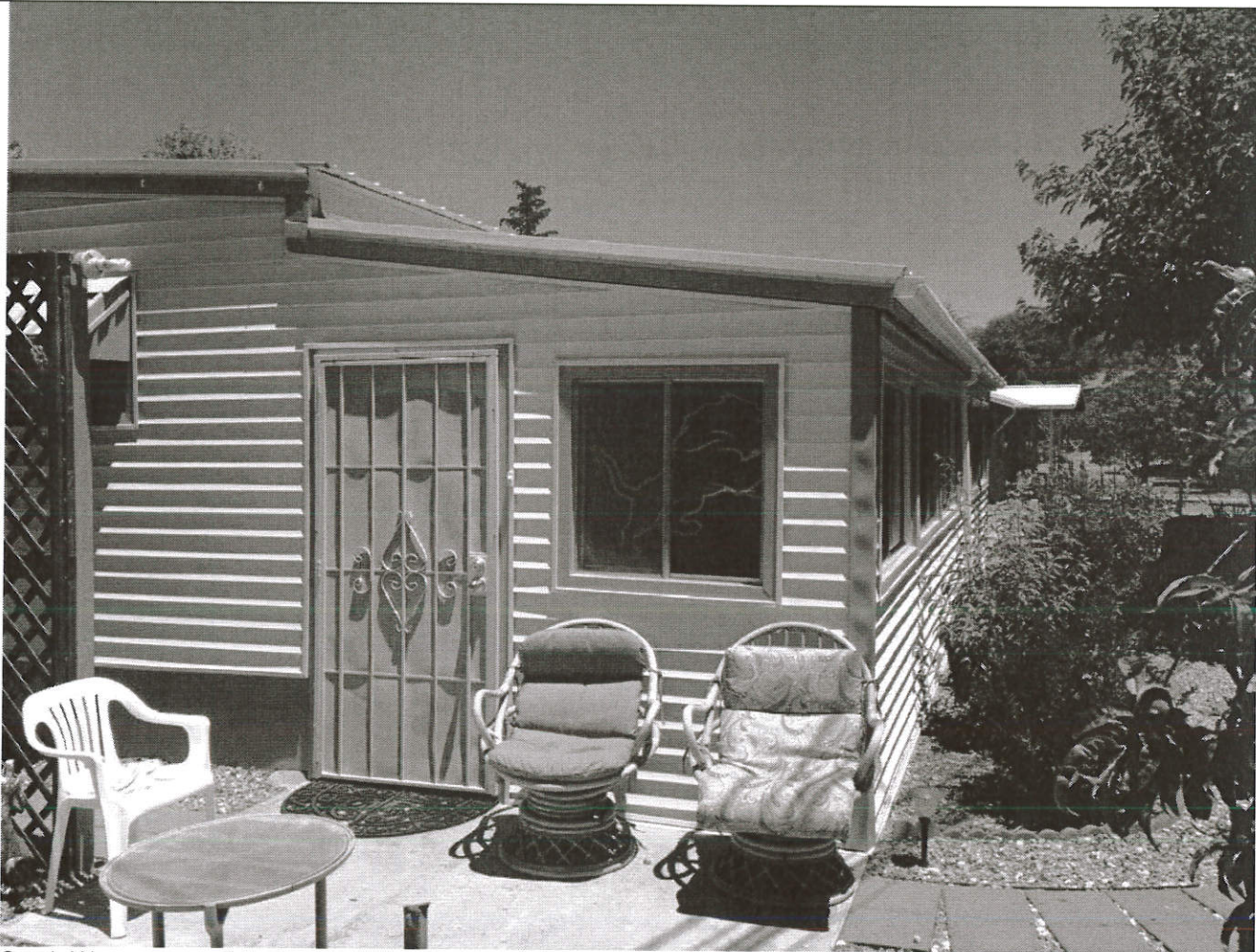
South West corner of the house. There is a crawlspace enclosed within stem walls (with one flood opening) on the north side of the house. South of that is a mobile home on supports with skirting around the base and a partial 11.6' section of stem wall, finished floor elevation 4757.16. The Arizona room is the next lower floor after this. Only the north part of the house has been included in the crawlspace square footage. Lag at deck or stairs is at deck.
