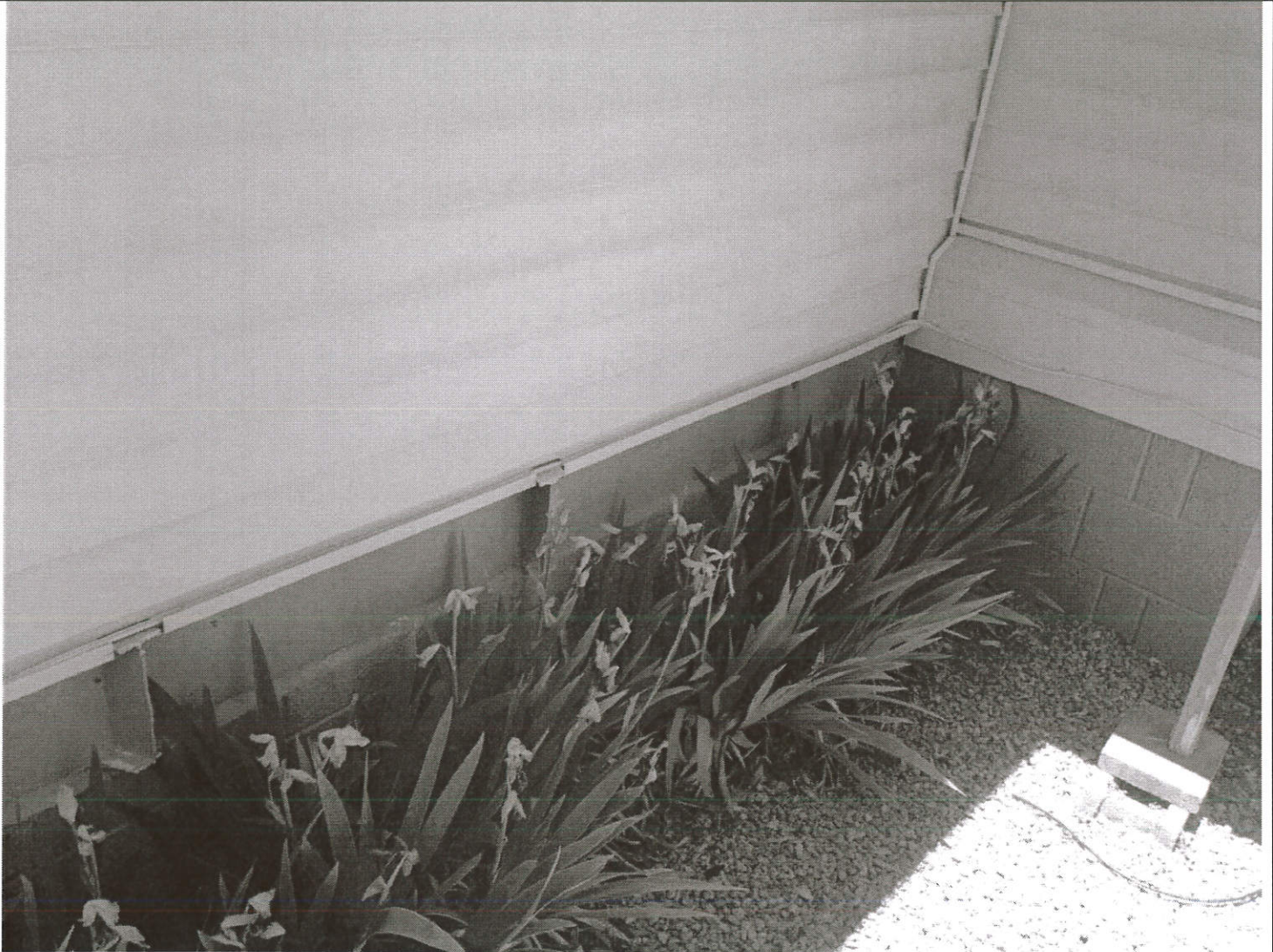
11.6' section of stem wall underneath mobile home on the East side.
