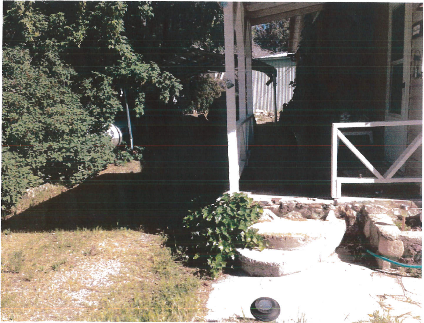
North East corner of the house (Stairs and Propane tank)
