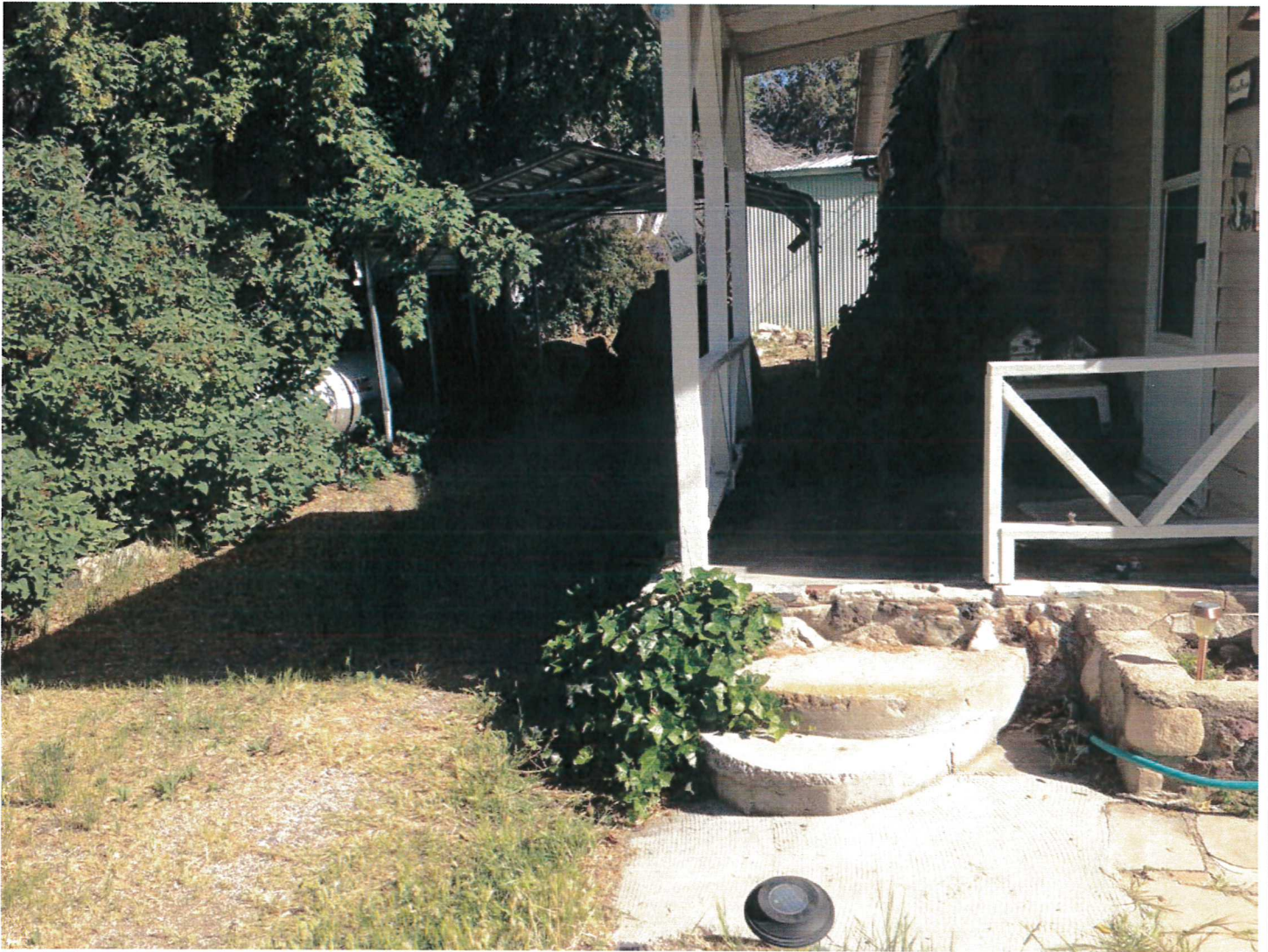
North East corner of the house (Stairs and Propane tank)
