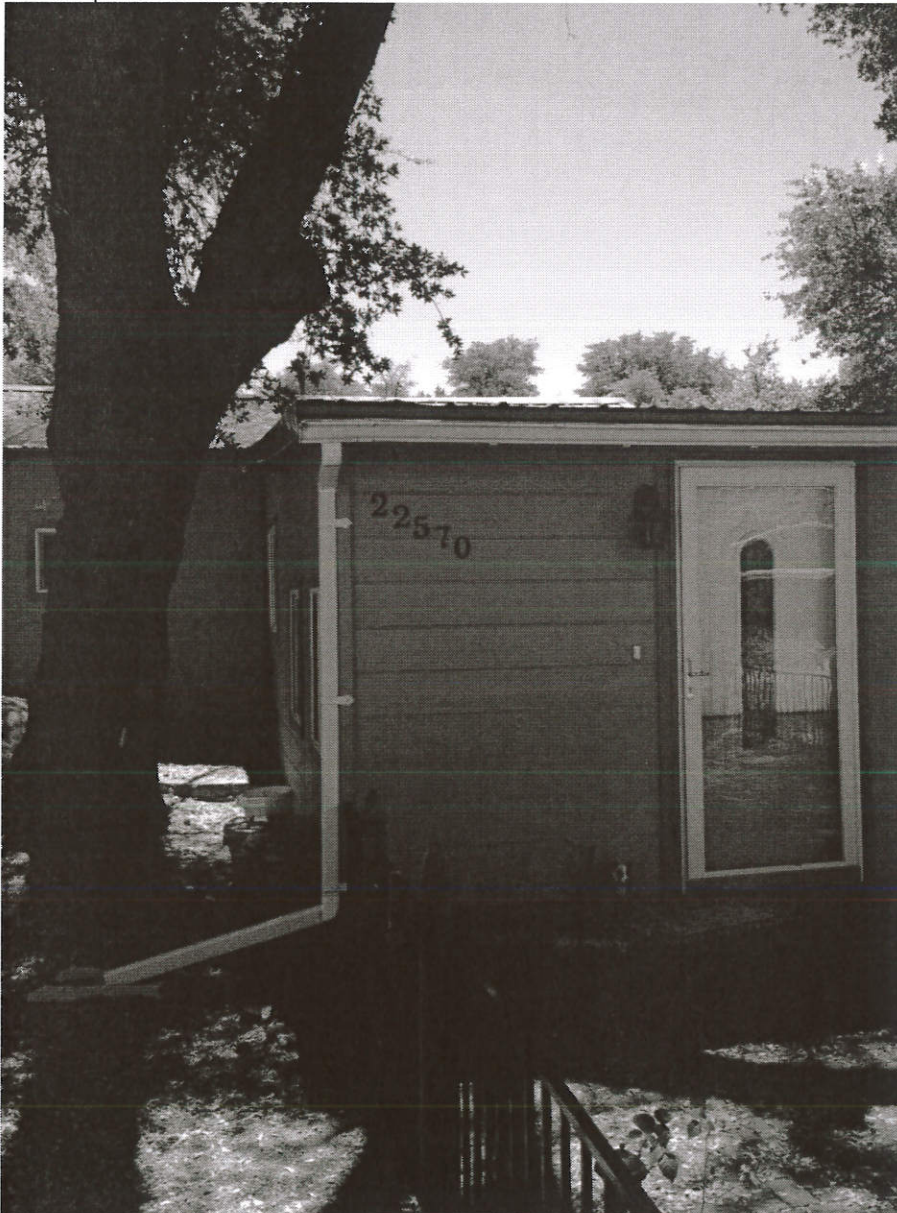
North side of house, Front, 05/29/15 (Bottom floor and stairs)
