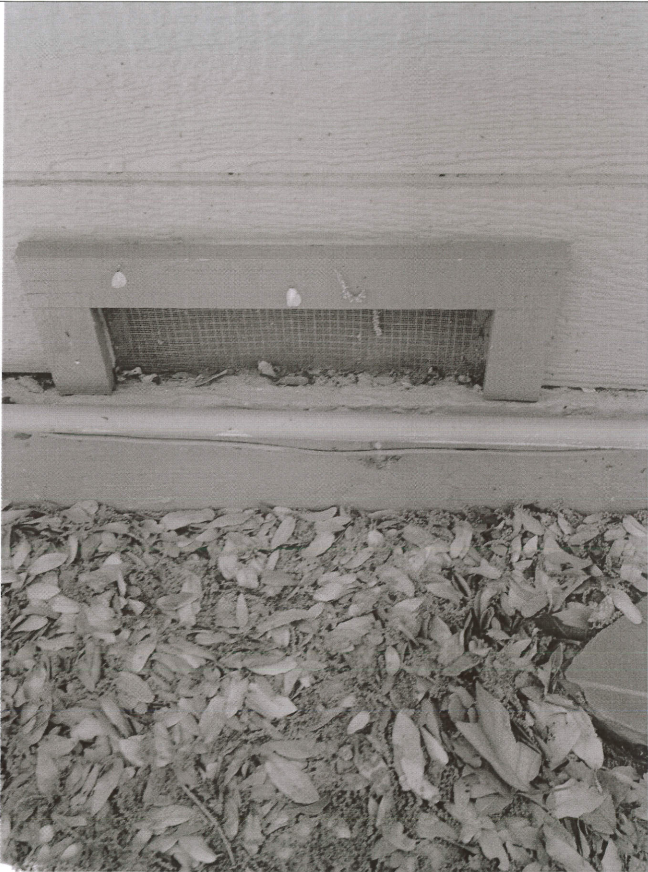
Flood opening on East side of the house. Right side, 05/29/15
