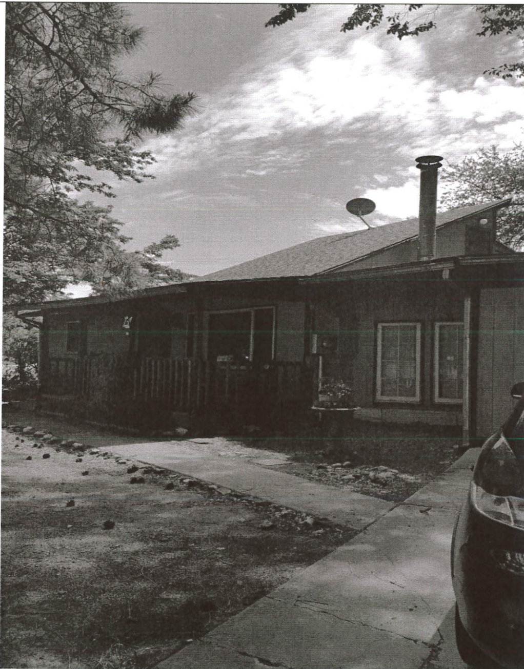
North side of house, front view, 06/08/15
