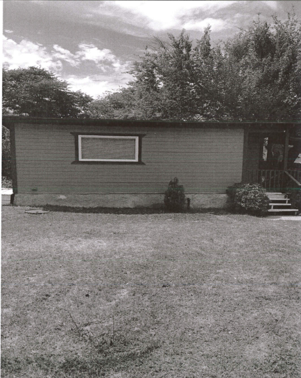
East side of house, right view, 06/08/15
