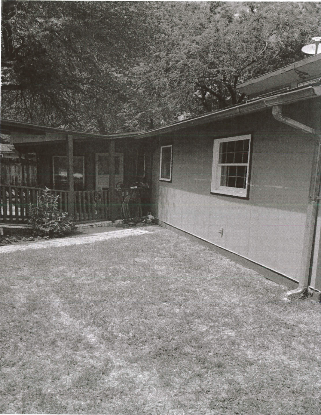
South side of house, rear view, 06/08/15 (Showing small Arizona room on the South West corner of house)
