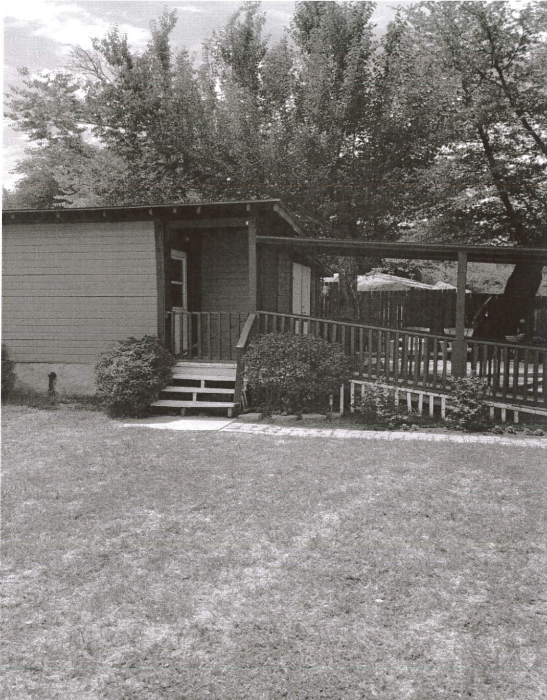
North side of house, front view, 06/08/15 (Showing stairs with opening underneath)
