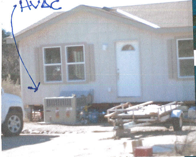
NORTH VIEW w/ HVAC
