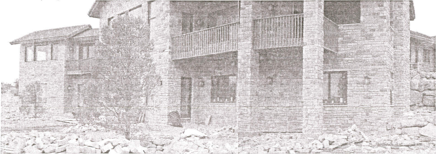
Rear View (East)
