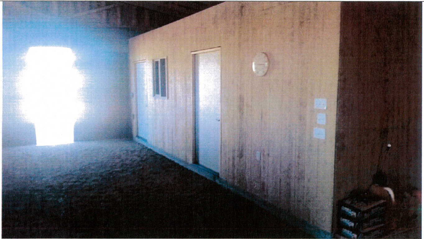
Interior of Barn
