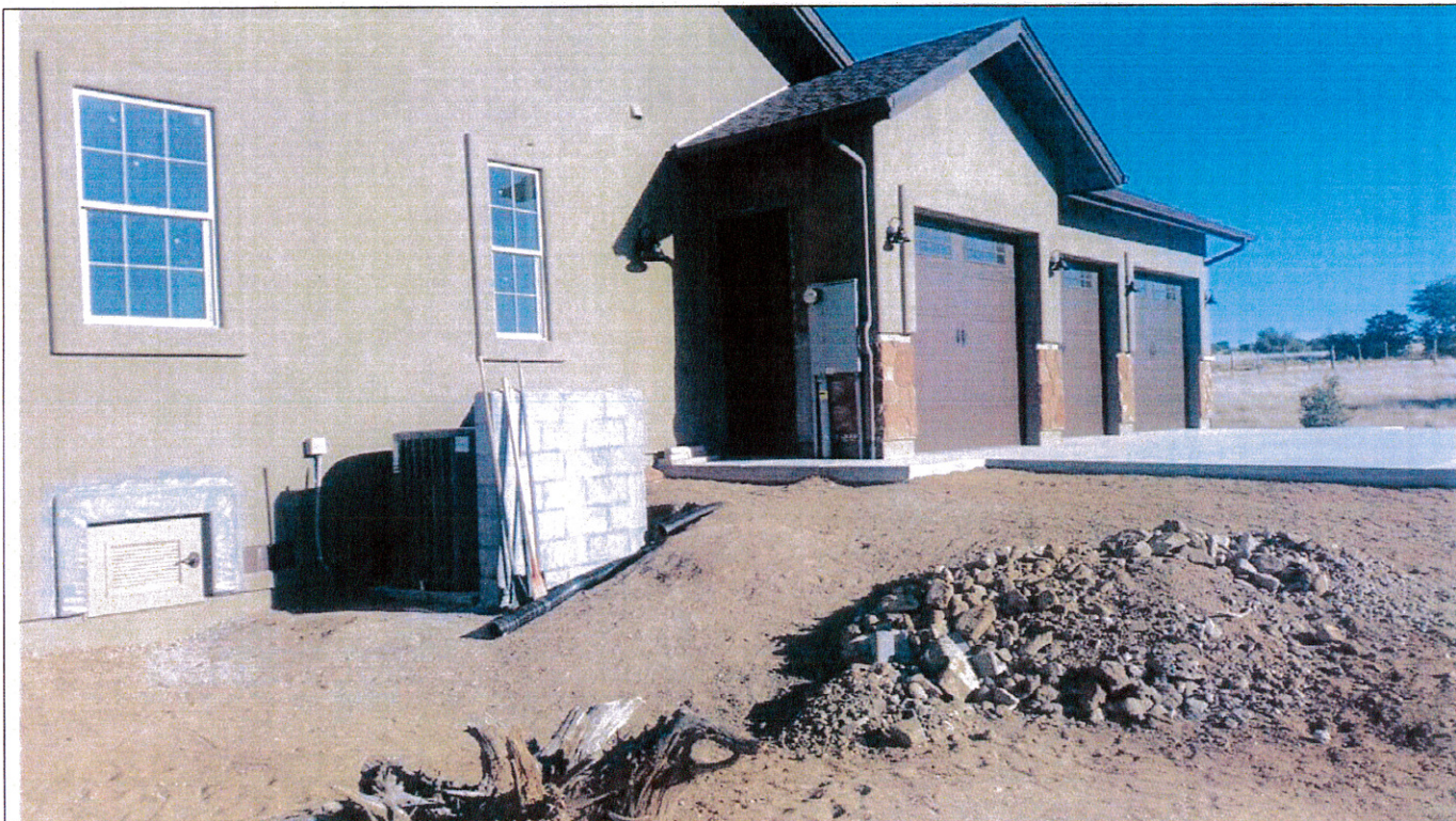
Northwest side of building, Lowest Equipment & Crawl space access
