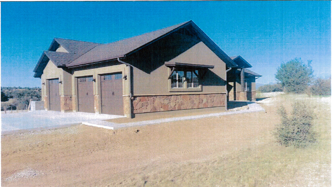
Southwest side of building, looking northeast
