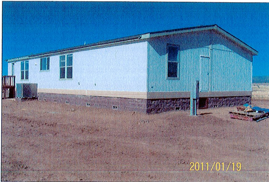
REAR VIEW (from left rear corner)
