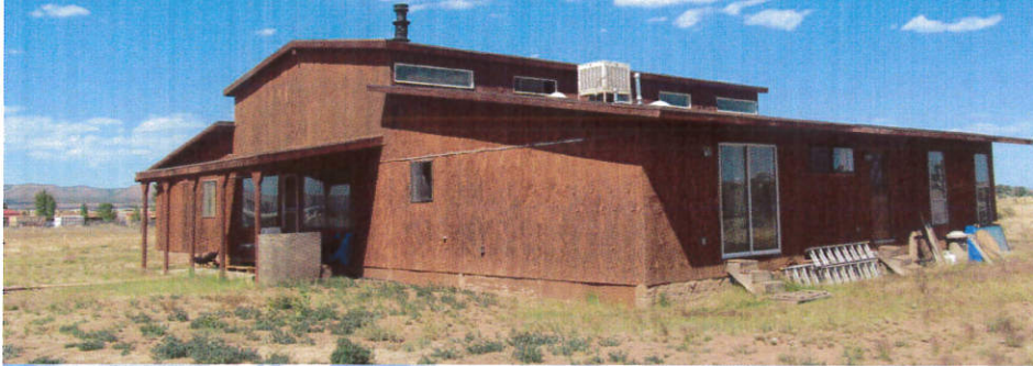
NORTH AND EAST SIDES OF HOUSE #1 LOOKING SOUTHWEST
