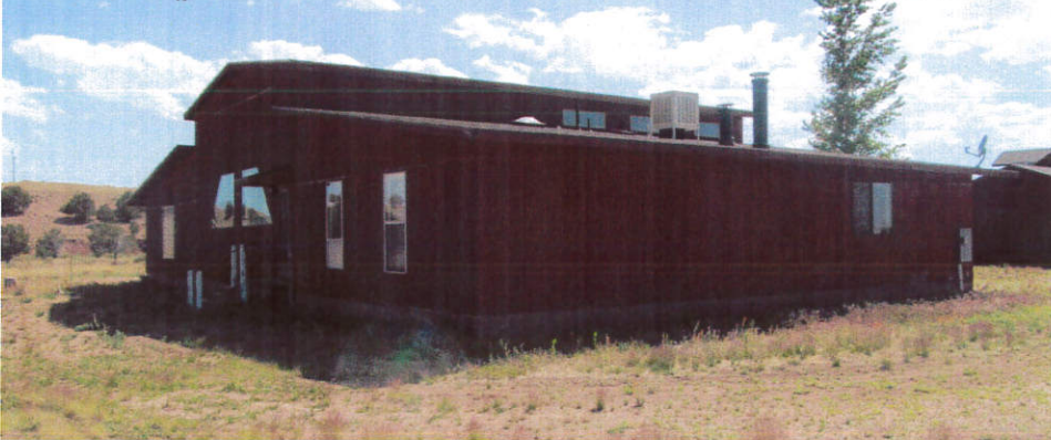
WEST AND SOUTH SIDE OF WELLHOUSE LOOKING NORTH
