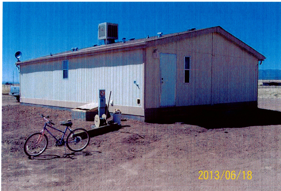
REAR OF HOME, FROM LEFT REAR CORNER
