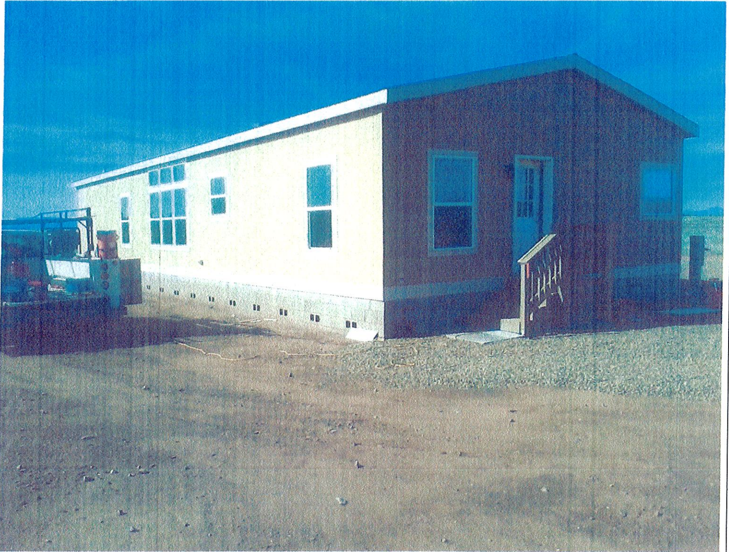
SOUTH SIDE-EAST END SHOWING ELECTRIC C2E AT RIGHT SIDE OF PHOTO
