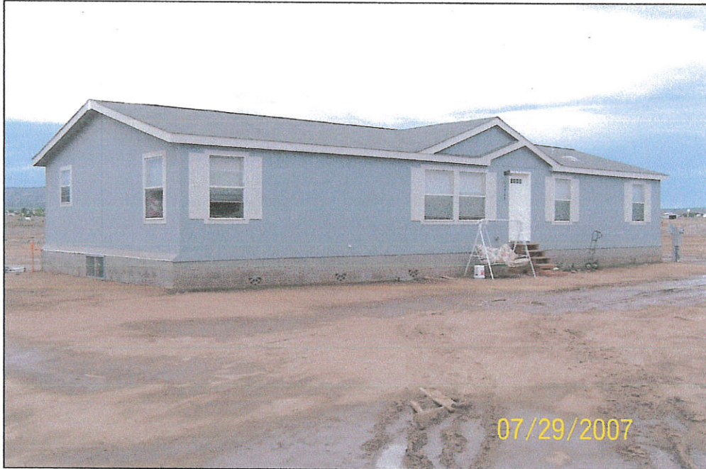
FRONT VIEW (from front left corner)
