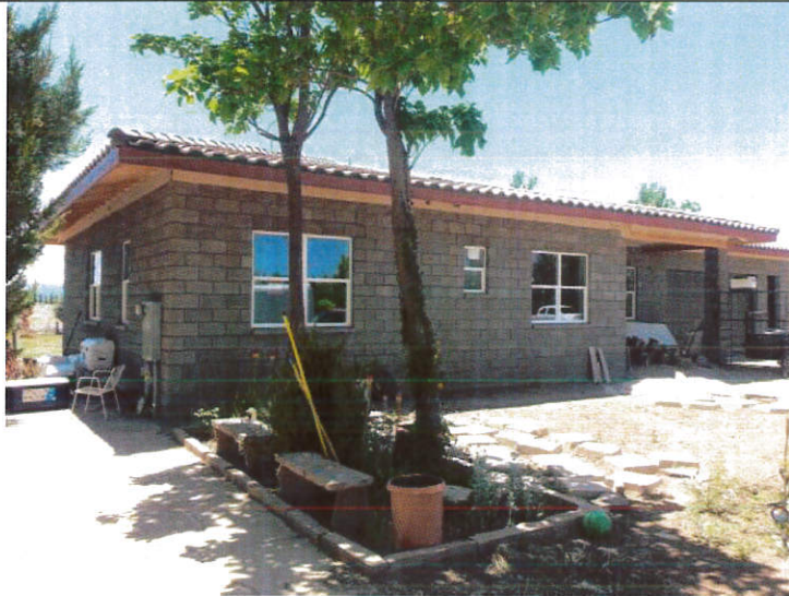
NORTH AND EAST SIDE BLDG. LOOKING SW 6-8-15
