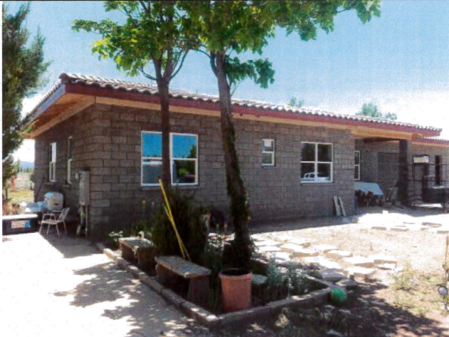
NORTH AND EAST SIDE BLDG. LOOKING SW 6-8-15
