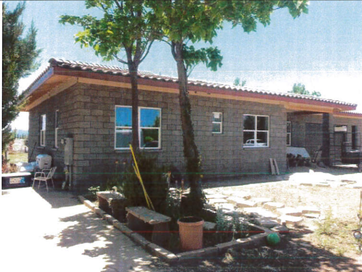
NORTH AND EAST SIDE BLDG. LOOKING SW 6-8-15
