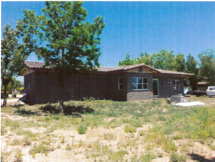
SOUTH AND WEST SIDE OF BLDG LOOKING NE 6-8-15
