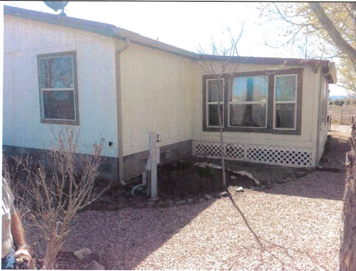
DECK, LOOKING WEST 4-6-16
