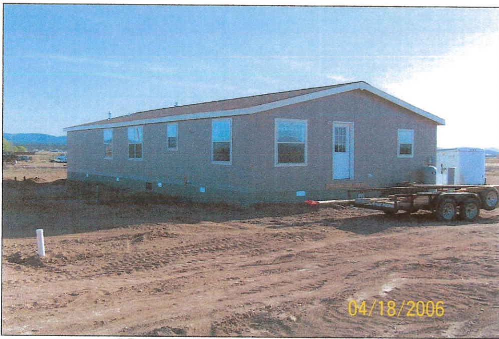
REAR VIEW (FROM LEFT REAR CORNER)
