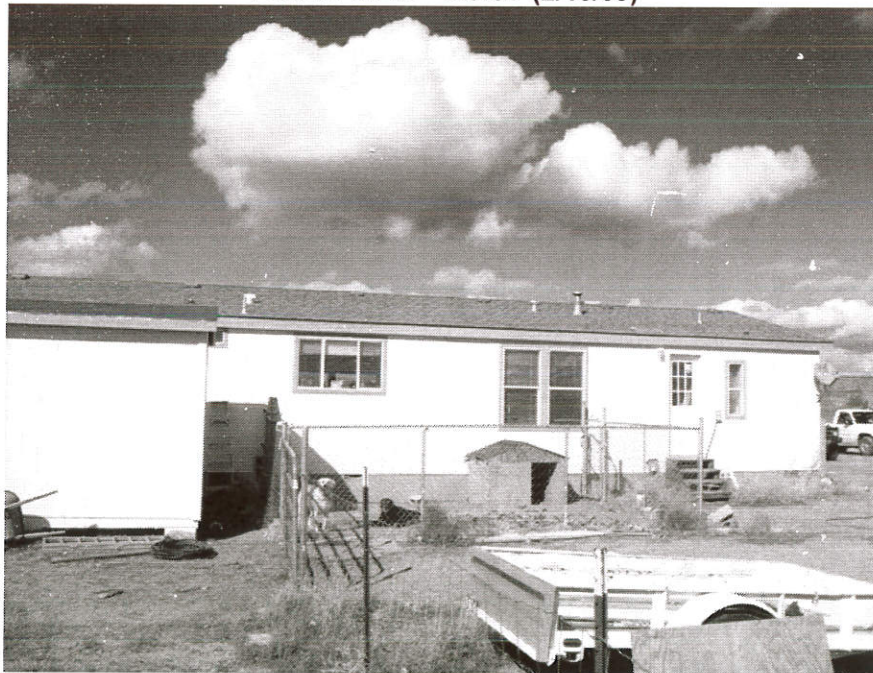
REAR VIEW – South (2/18/09)
