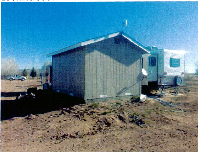
WEST AND SOUTH END SHED, LOOKING NORTHEAST TOWARDS ROAD 4-8-2014
