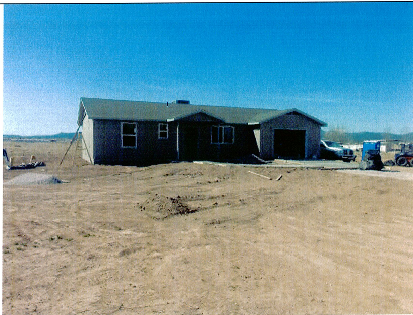
FRONT AND EAST END LOOKING SOUTH
