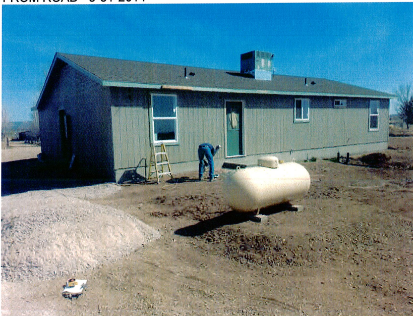
REAR AND WEST END LOOKING NORTH
