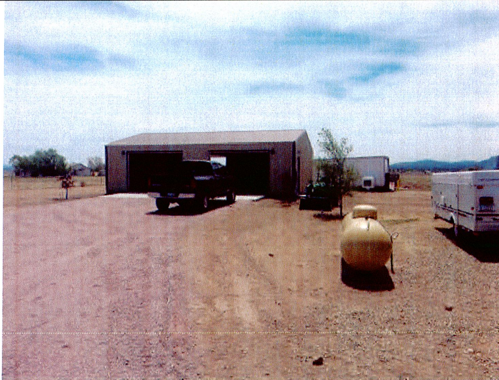
FRONT AND WEST SIDE GARAGE LOOKING
