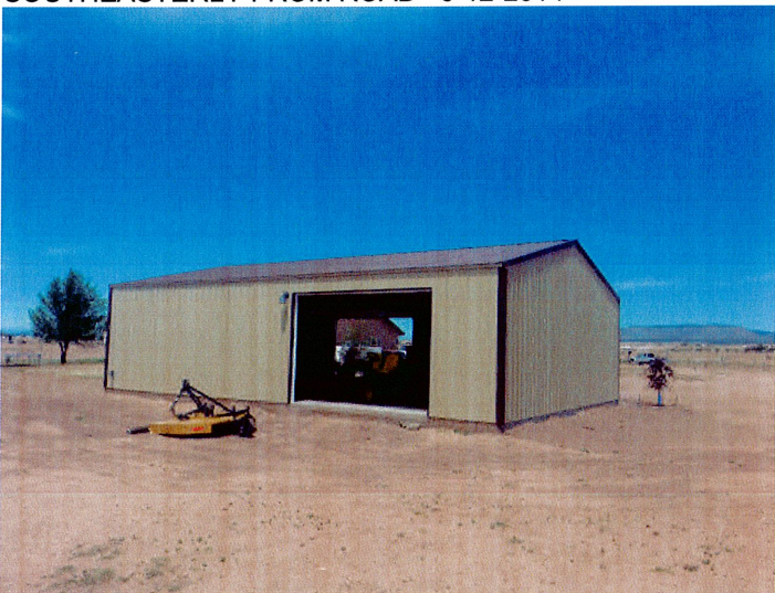
REAR AND EAST SIDE OF GARAGE. LOOKING
