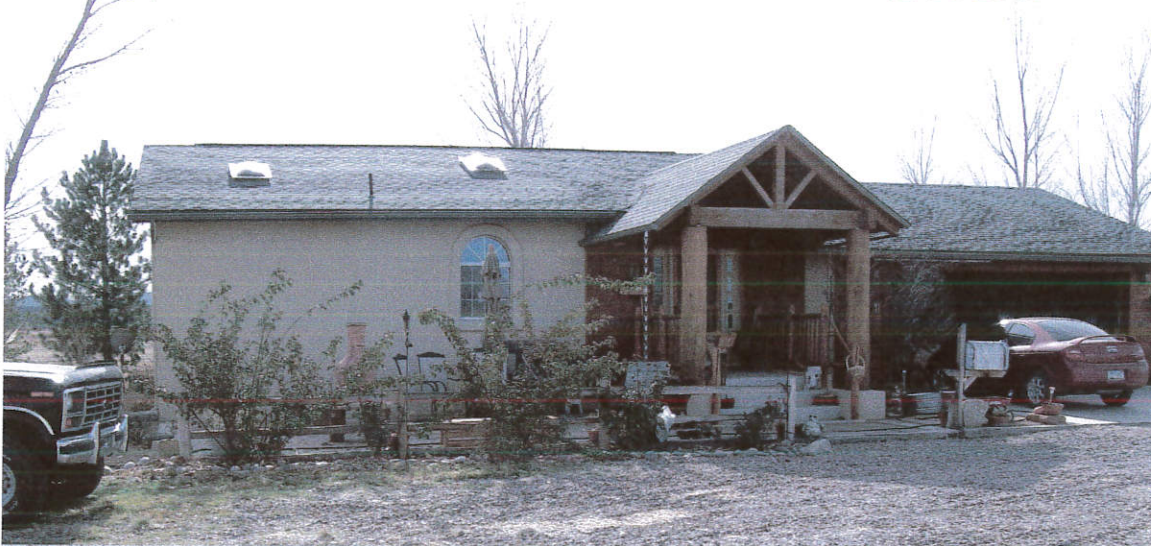
SOUTHWEST CORNER, LOOKING NORTHEAST
