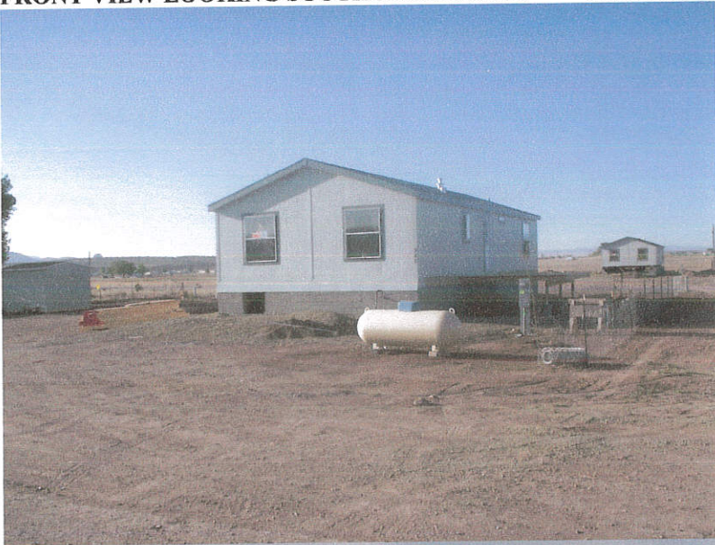
FRONT VIEW LOOKING SOUTH FROM ROAD PHOTOS TAKEN 5-15-2006
