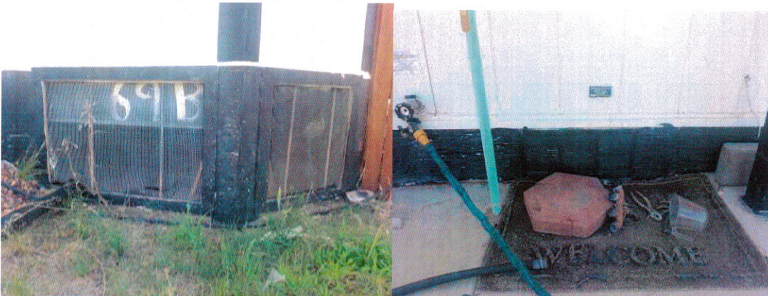
SCREEN VENTS AT NORTHWEST CORNER AND REAR HOUSE 8-25-15
