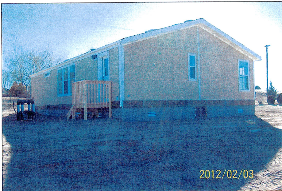
REAR VIEW (from left rear corner)
