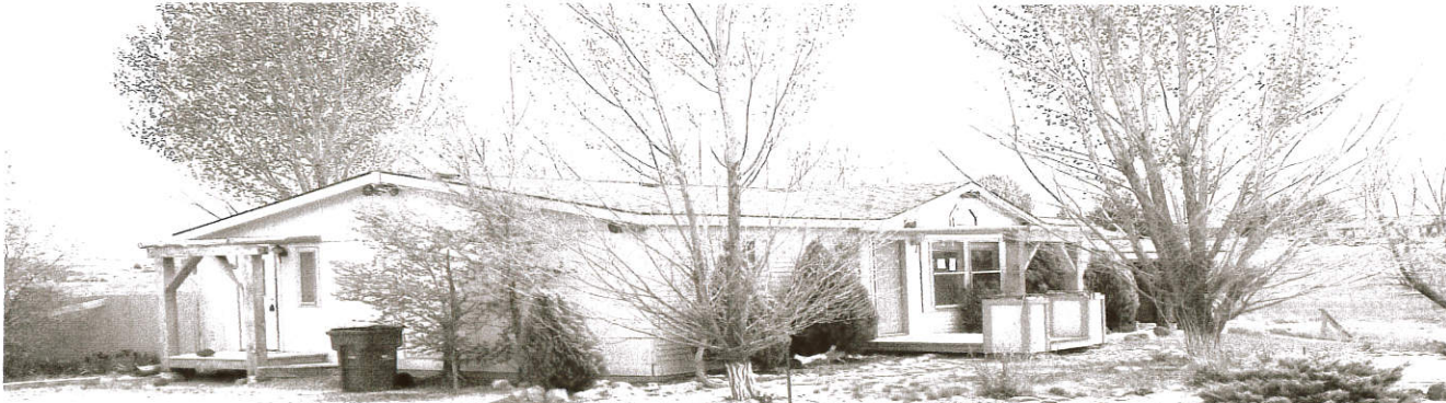
FRONT LOOKING SOUTHEAST FROM STREET 5-2-2009
