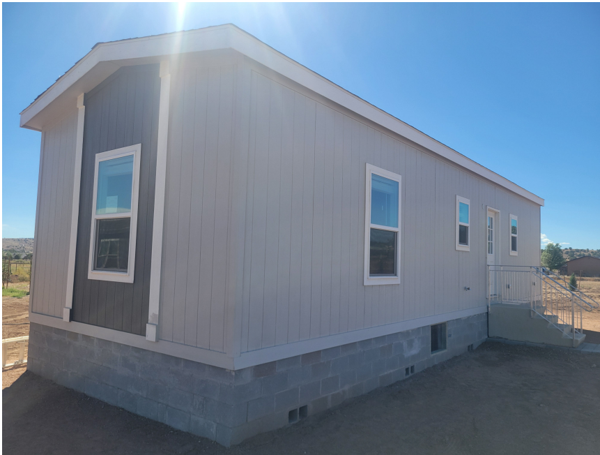
Photo One Caption: NW CORNER LOOKING SE FROM TATANKA CIRCLE 9-10-2025
