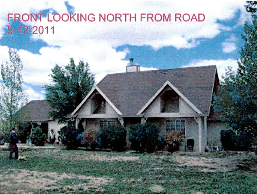
FRONT AND EAST SIDE LOOKING NORTH FROM ROAD 5-12-2011
