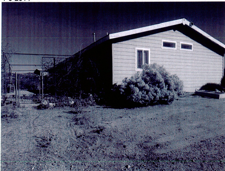
REAR AND SOUTH END LOOKING NORTHEAST
