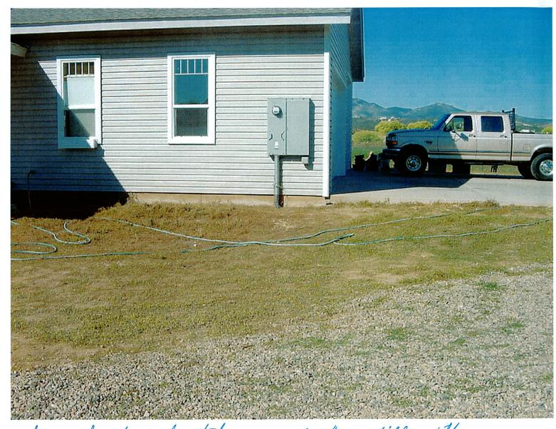
home has hen elevated on approx 18" of fill with stemuall above + FFE approx 8-10" above fill so no openings where necessary
