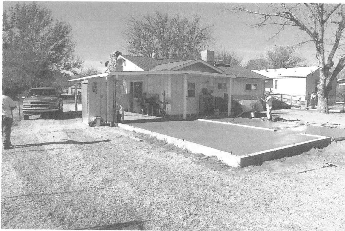
NEW CONCRETE PAD FOR GARAGE ADDITION
